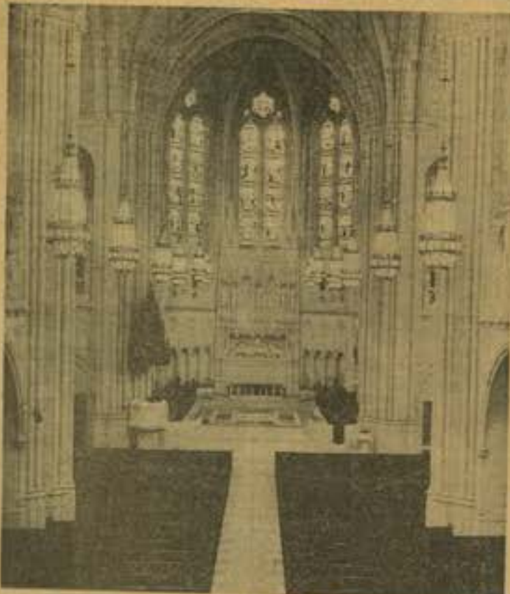
Majestic beauty—enveloped in quiet light! A view of the interior of the new East Liberty Presbyterian Church, whose pillars rise 74 feet to great vaulted arches, illumined by high stained glass windows. In the chancel at the front may be glimpsed John Angel's sculptured interpretation of the "Last Supper."
